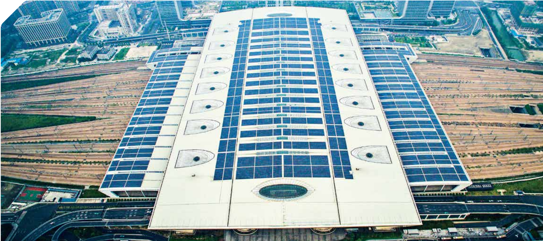
10MW 屋顶光伏电站 Hangzhou East Railway Station Hangzhou, Zhejiang Province, China
