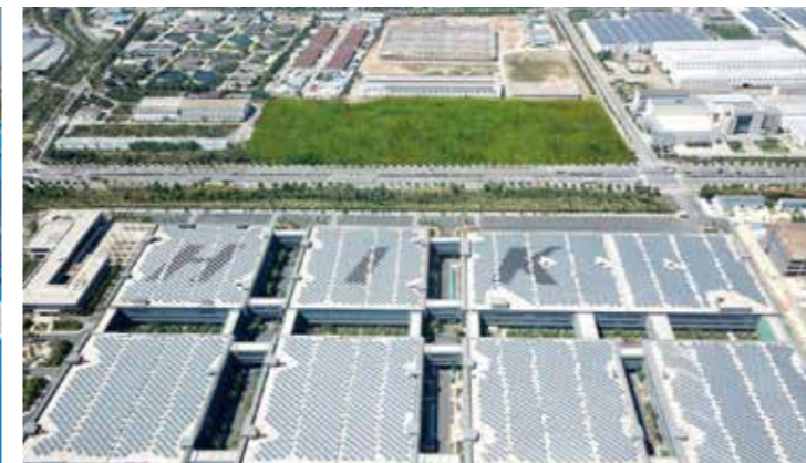
10MW Hikvision Rooftop Project Hangzhou, Zhejiang Province, China
