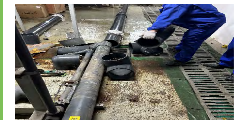
Installation of ultrafiltration drain
